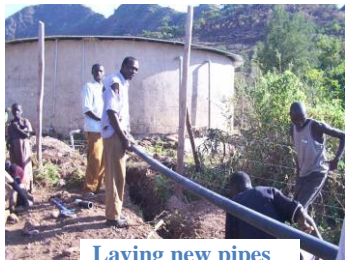
Laying new pipes
